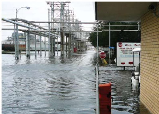
INVISTA's plant in Orange, Texas, was heavily damaged by Hurricane Ike and remains shut down.
