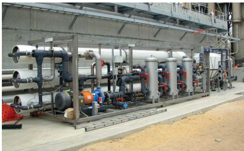
A single MegaMagnum® unit from KMS, such as this installation in Australia, can produce 500,000 gallons of reusable water per day.
