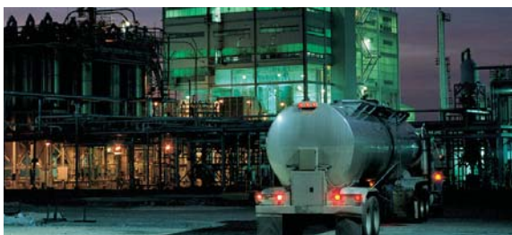
Odessa, Texas – This polymer plant is included in the FHR acquisition.
