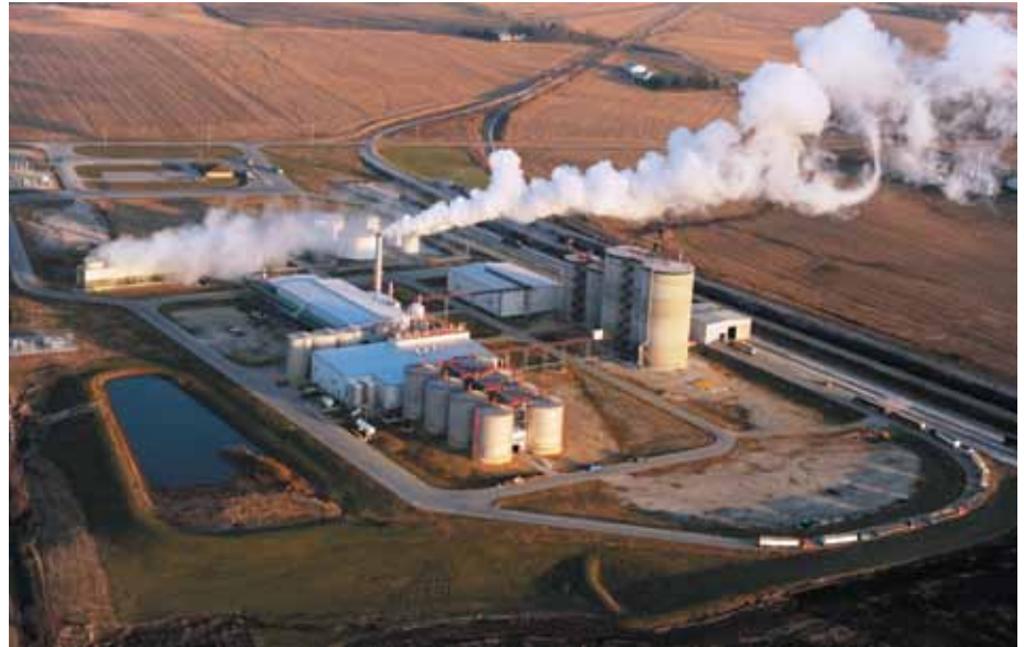
Built in 2008, this second-generation ethanol plant in Menlo, Iowa, is one of two purchased by FHR in September.
