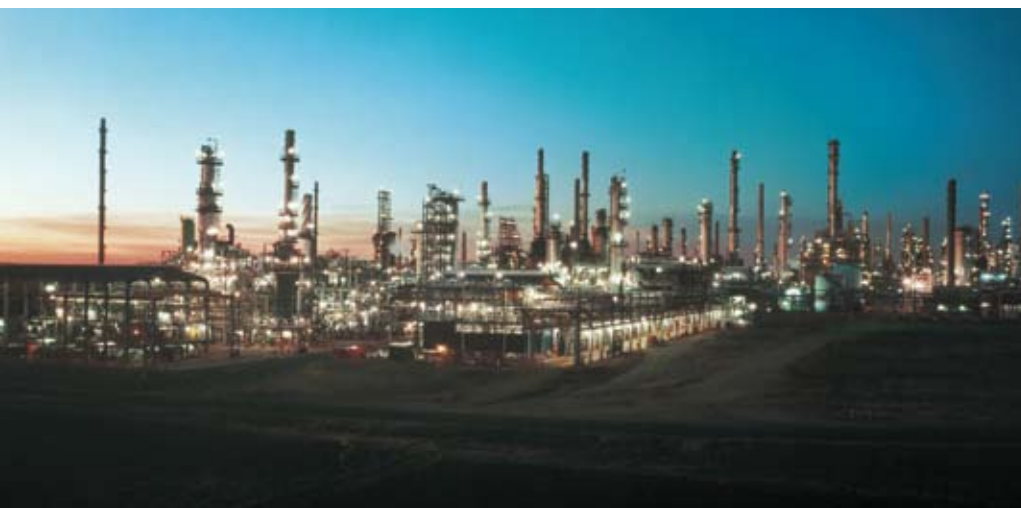
Pine Bend Refinery in Minnesota was designed to process high-carbon Canadian crude.
